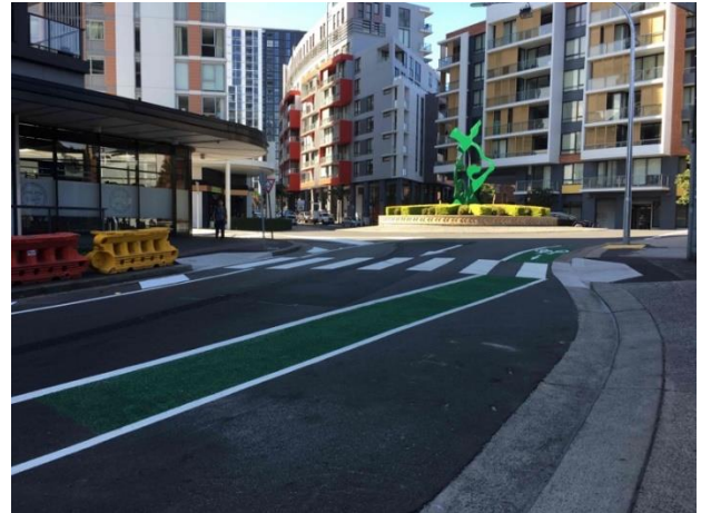
Photo above: new line marking on Arncliffe St
